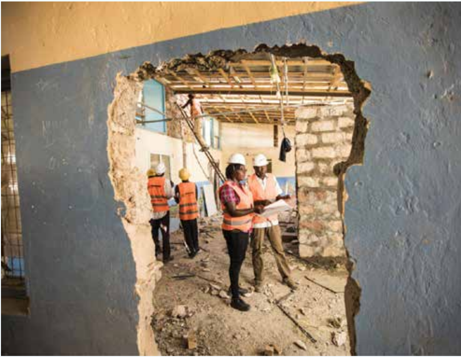
UNOPS engineers inspect a construction site in Turkana, Kenya
